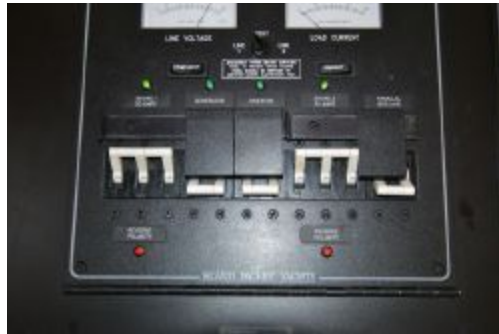
Shore/Gen selector and start panel
