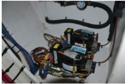
Two independent refrigeration units
