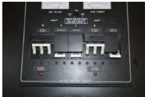
Shore/Gen selector and start panel
