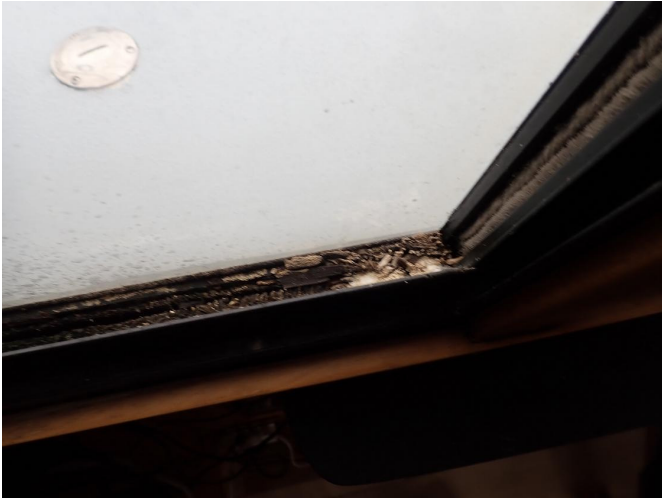
Felt tracks deterioration, slider windows
