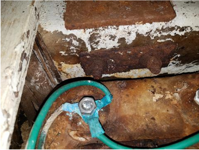
Heavy corrosion noted for most bonding wire connections
