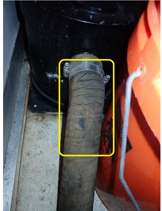
Generator exhaust hose age cracking at waterlift
