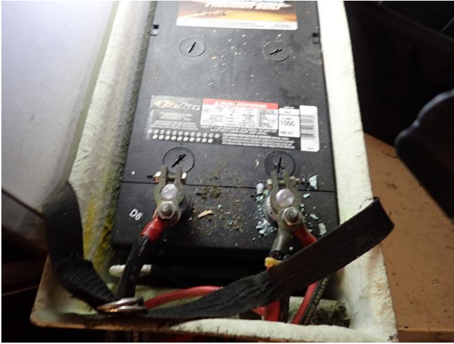
D6 (April 2016) date code for generator lead acid battery
